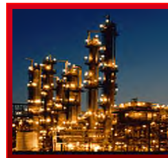
Scotford Refinery (Shell only)
